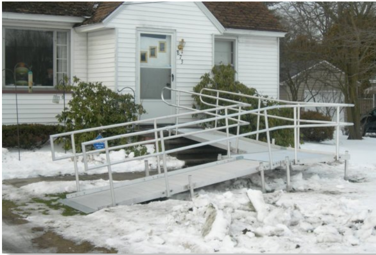
Aluminium Ramp Installed
