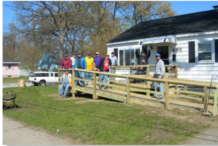
By contrast, this is one of the crew's wooden ramps
